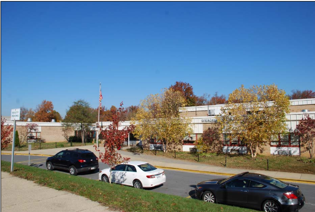
Figure 8. Greenbelt Site, Springhill Elementary School
