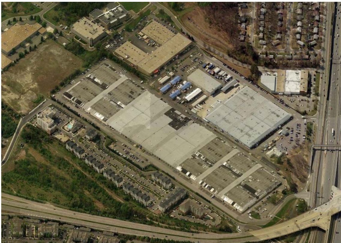
Figure 2. GSA Warehouse Property, looking south
