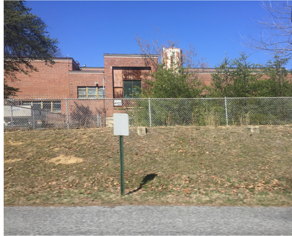
5 Supersonic Wind Tunnel Building
