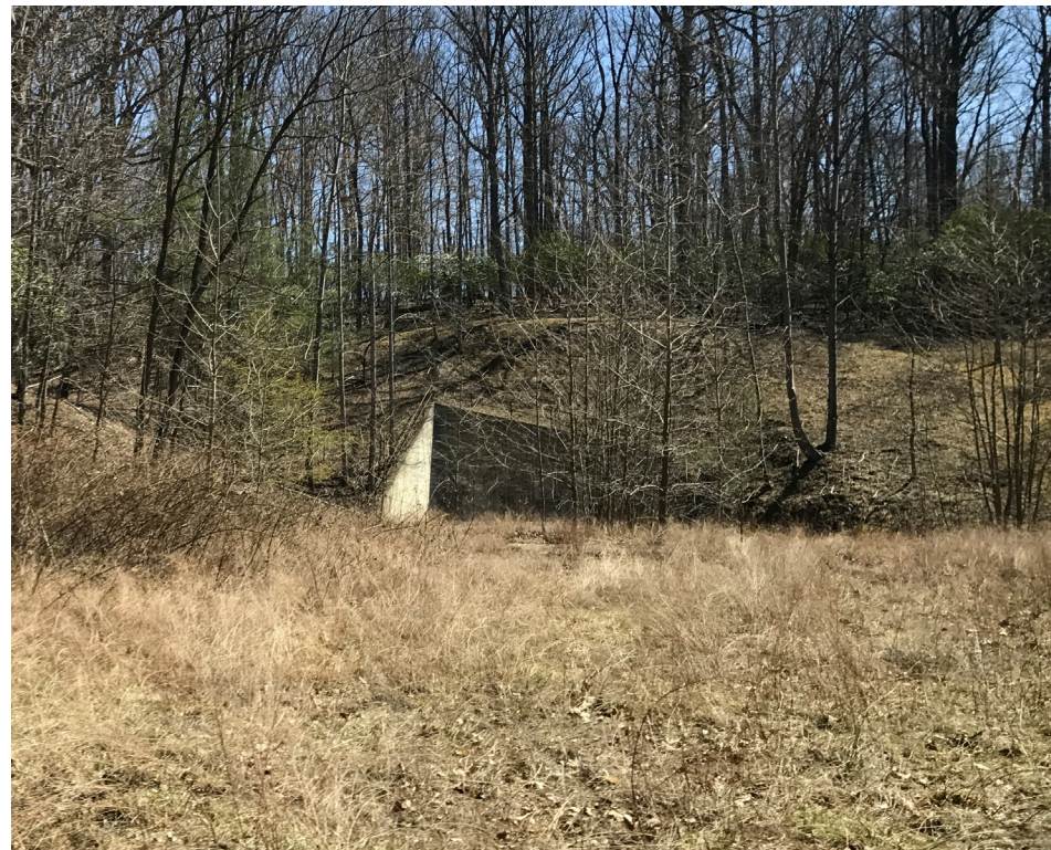
2 Concrete retaining wall near Paint Branch
