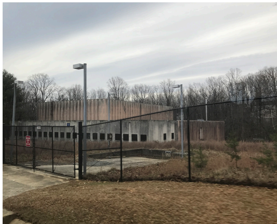
1 Former Defense Nuclear Agency Casino Facility
