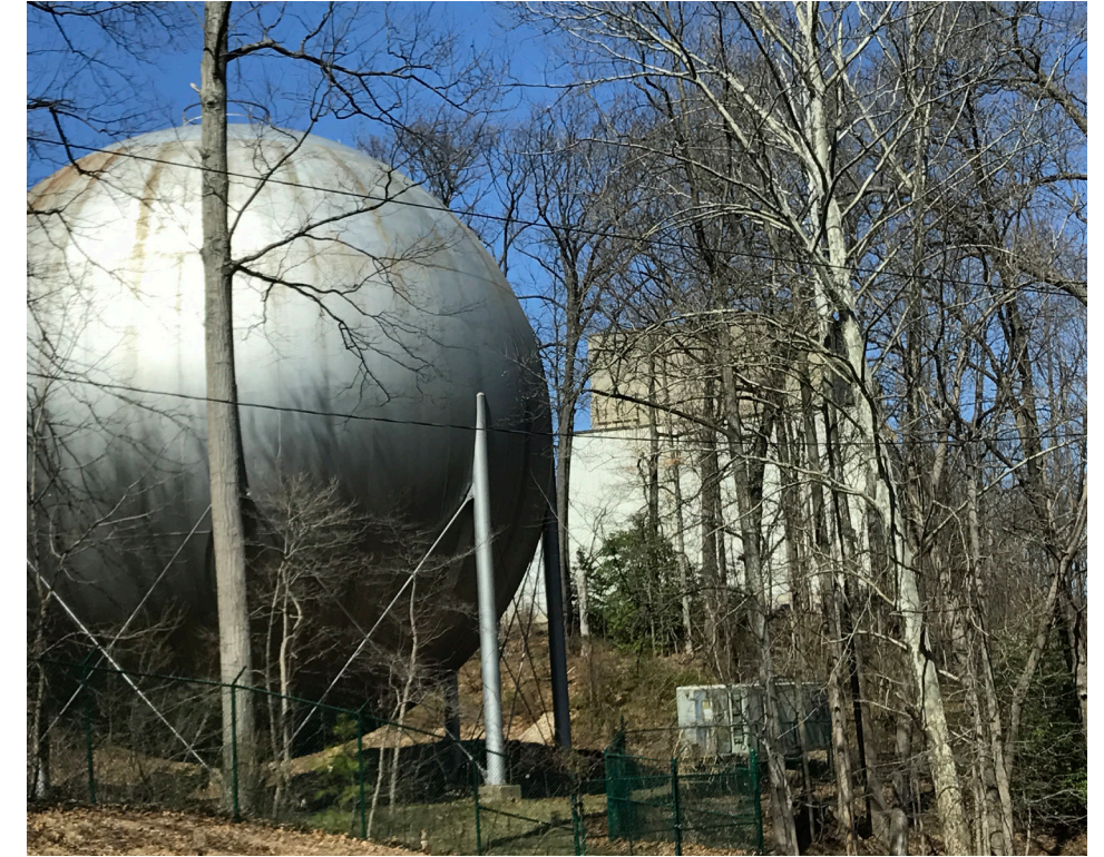
6 Vacuum Sphere and Hydroballistics Tank Building
