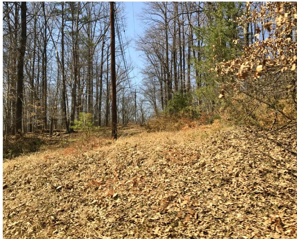
1 View of existing overhead power lines and clearing
