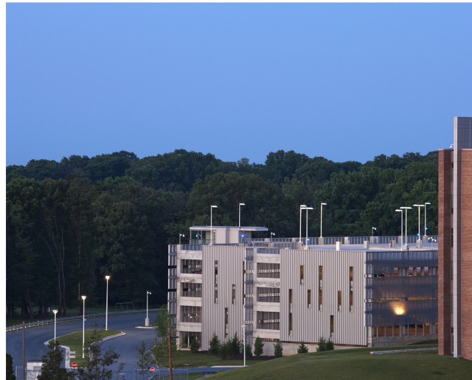
8 Southwest Parking Garage
