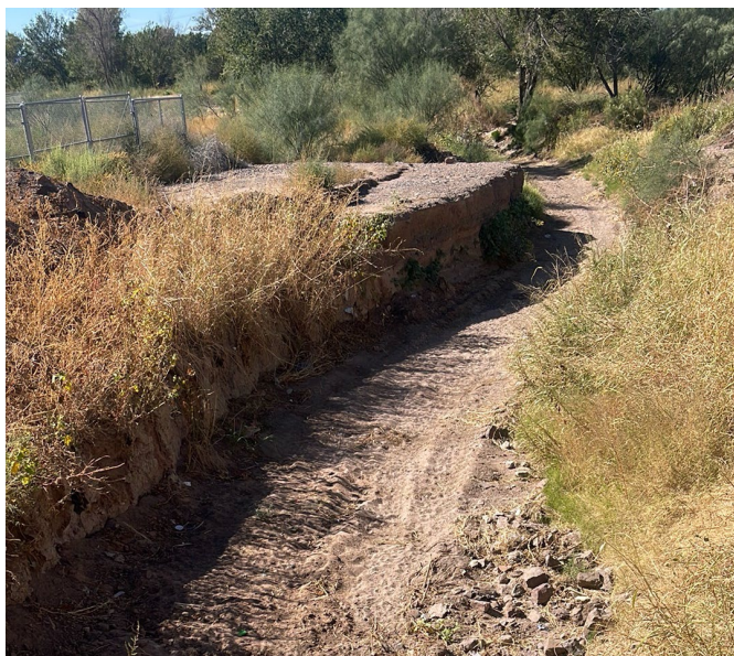
Figure 3.5-2. Erosion and Scour of Channel Banks within Unnamed Wash, North Section of Project Area, facing West
