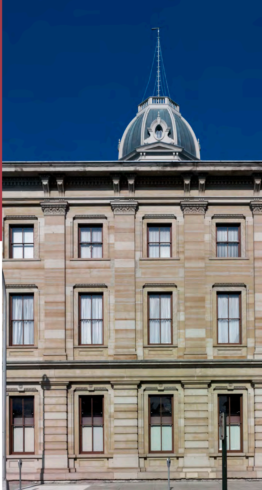
Federal Building and U.S. Courthouse Port Huron, MI
