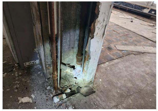
3rd Floor: Storm stack. Portions of the existing piping were replaced with PVC piping as part of emergency repairs performed to alleviate building flooding.
