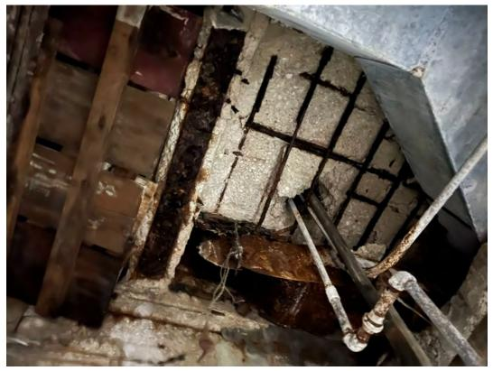
Upper basement slab from below: Area with exposed and corroded rebar and steel
