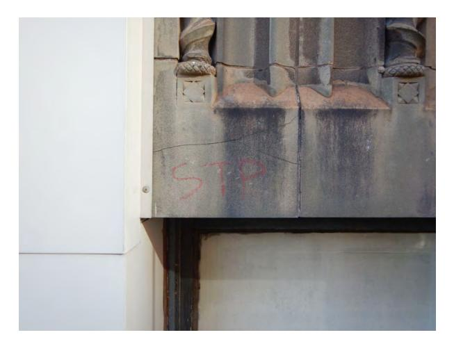
Terra cotta spandrel with cracked window head unit
