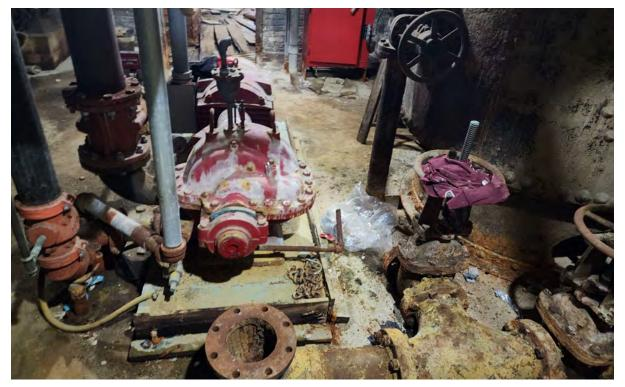
Basement Level: Fire pump, fire pump controller, and damaged abandoned FP piping
