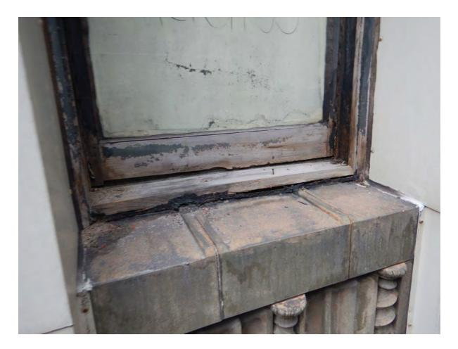
Typical deteriorated wood window with failed coatings, sealants and glazing
