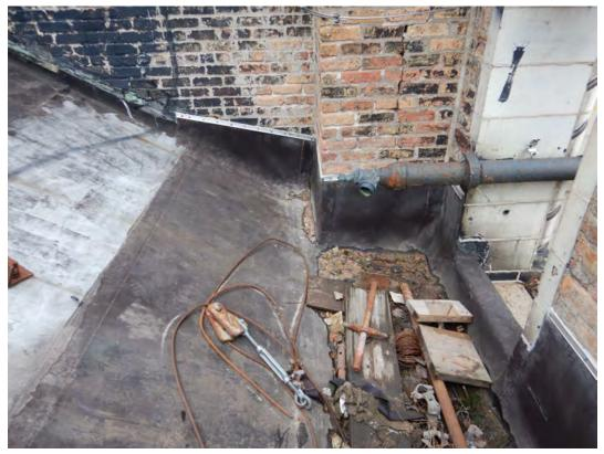
Northwest corner of roof, the only roof drain was buried under debris
