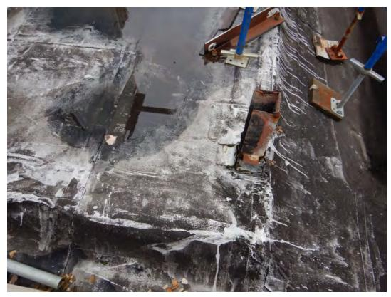
Failed roofing membrane and ponding water on upper flat roof
