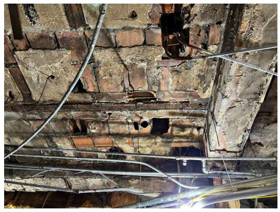
Ground Level floor from below: Isolated damage to clay tile floor system
