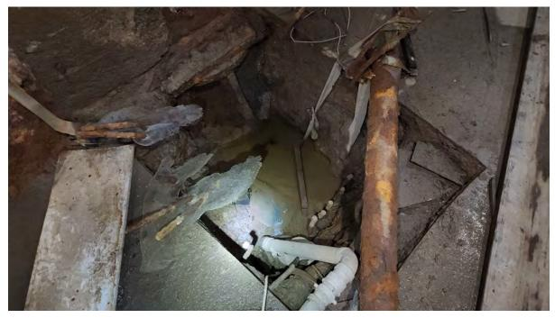
Basement Level: Floor slab has been cut and a temporary pump pit has been created to mitigate basement flooding by collecting water. A simplex pump was put into the pit to pump out the water.
