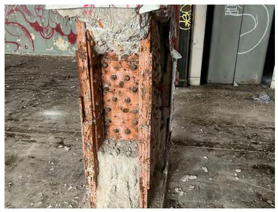
Superstructure: Previously removed concrete encasement on steel column
