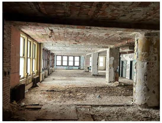
Superstructure: Typical upper floor layout and clay tile arch floor system, looking east
