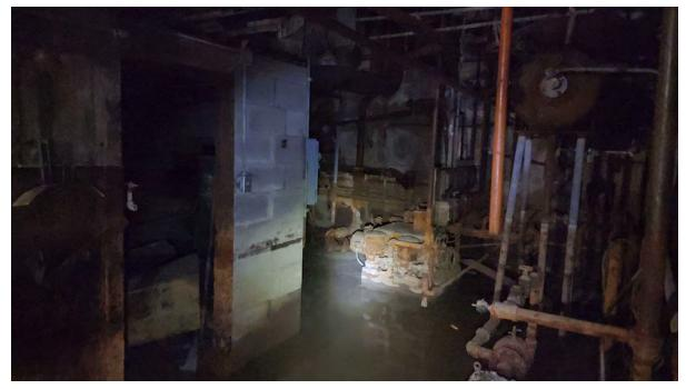
Basement Level: Mechanical and Plumbing equipment in flooded area of the basement. The water ponding is several inches deep.
