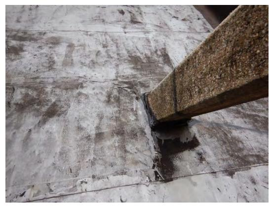
Failed roof membrane at parapet brace
