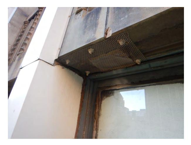
Continuous mullion clad in aluminum sheeting and spandrel unit
