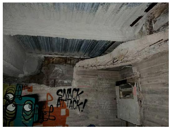
Ground Level slab from below: Vaulted slab on deck at east sidewalk
