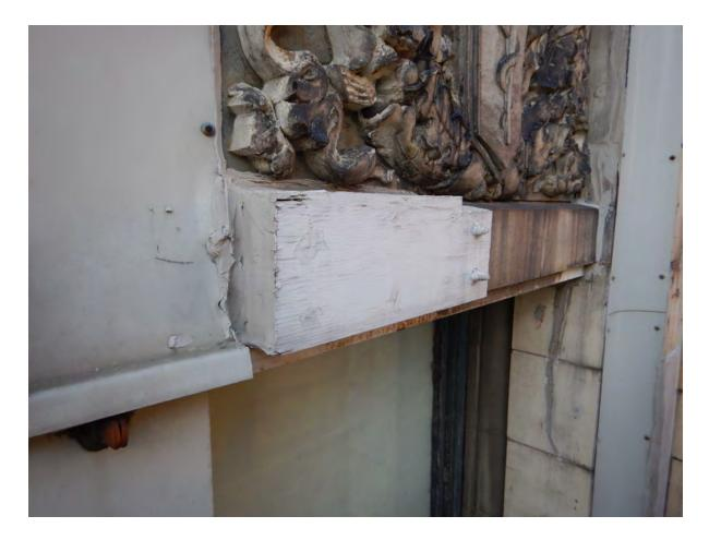
Terra cotta spandrel unit with channel beneath and cracked terra cotta jamb units
