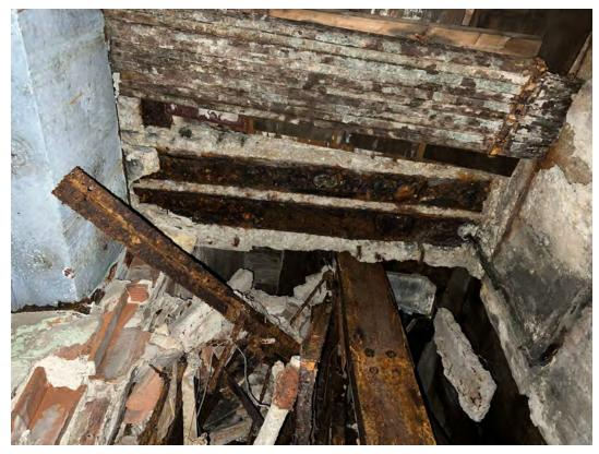
Upper basement slab from below: Corroded steel beams with missing cover above elevator pit
