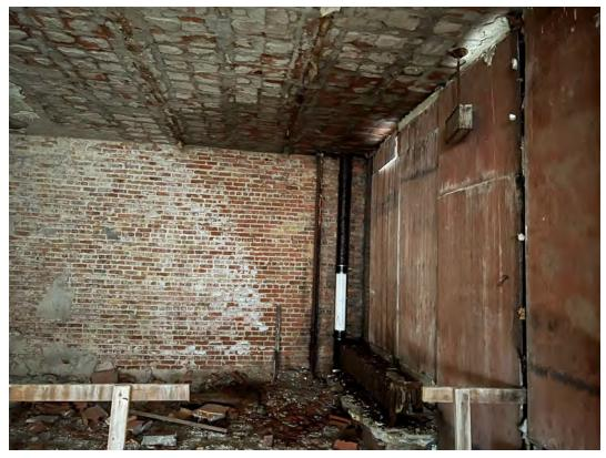
Superstructure: Observed water infiltration at northwest corner of slab typical Levels 7 - Roof
