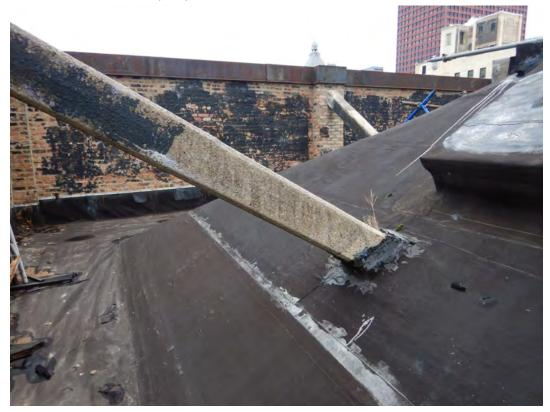
Vegetation growing out of diagonal brace to roof membrane juncture
