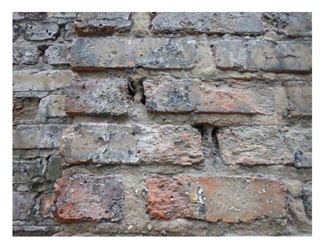
Weathered brick masonry and mortar joints
