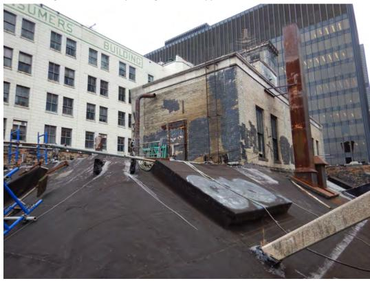
Sloped section of roof with roof covered skylight, penthouse in background
