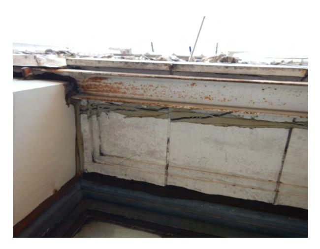
Terra cotta spandrel unit with channel beneath and cracked terra cotta units
