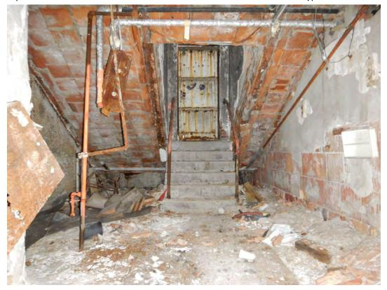
Roof framing: Clay tile encased roof framing, photo take from attic
