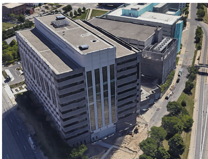
Aerial view of 985 Michigan showing the main building and parking garage. Cooling towers are adjacent to the parking garage.
