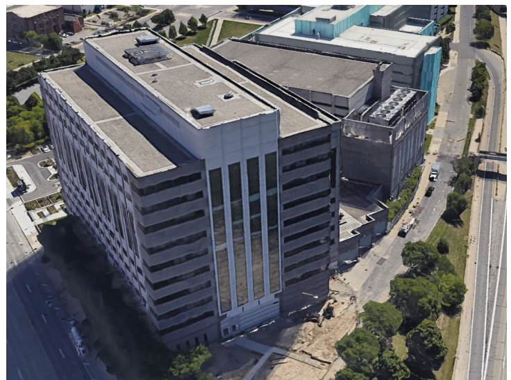
Aerial view of 985 Michigan showing the main building and parking garage. Cooling towers are adjacent to the parking garage.
