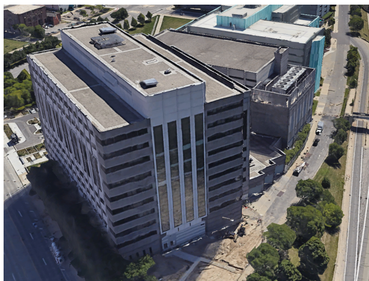
Aerial view of 985 Michigan showing the main building and parking garage. Cooling towers are adjacent to the parking garage.
