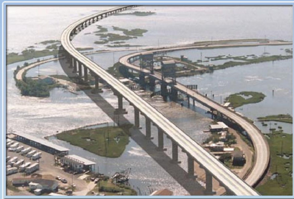
Adaptation Possibilities for Coastal Infrastructure
