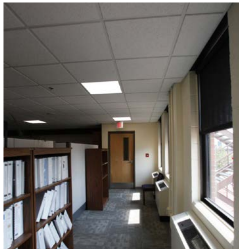
Figure 21 Image of Building 1219, Open Office Perimeter
