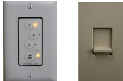
Figure 39 Images of Building 9447 and 9420, Conference Room Control Interfaces
