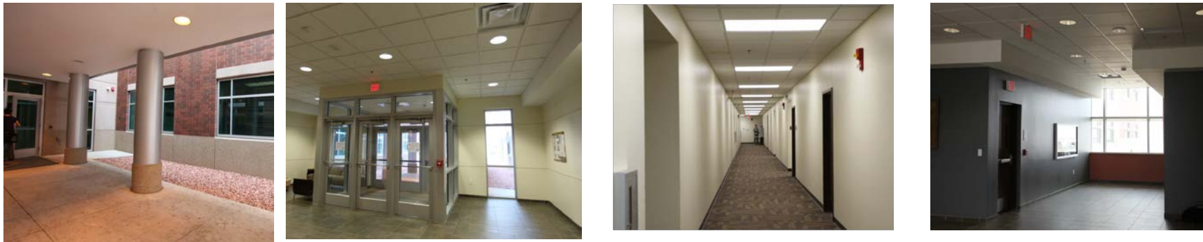
Figure 33 Images of Building 9420, Shared Spaces
