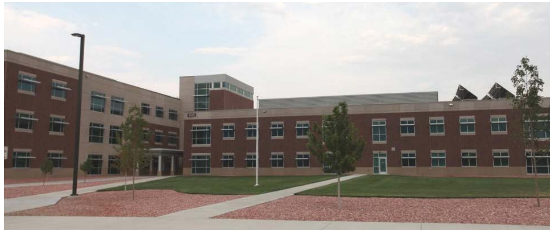
Figure 32 Image of Building 9420, West Façade
