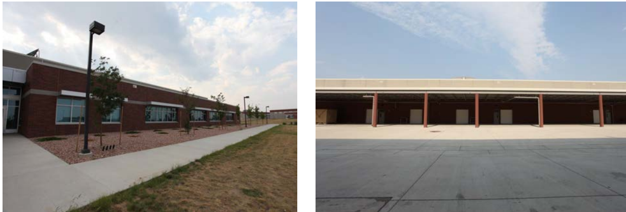
Figure 25 Image of Building 9447, Primary Façades
