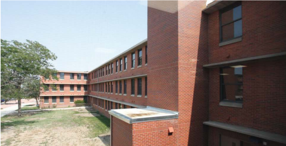
Figure 14 Image of Building 1219, North Façade
