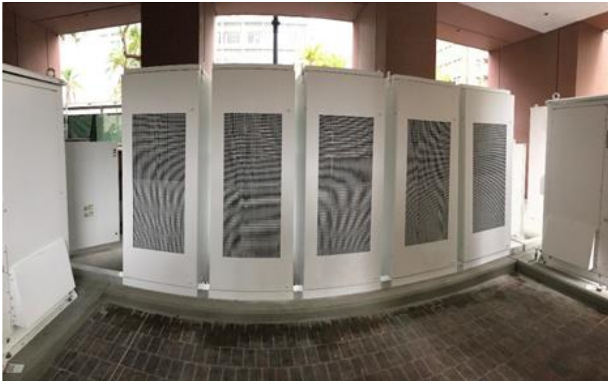
Image: GSA: Schwartz Federal Building and Courthouse
