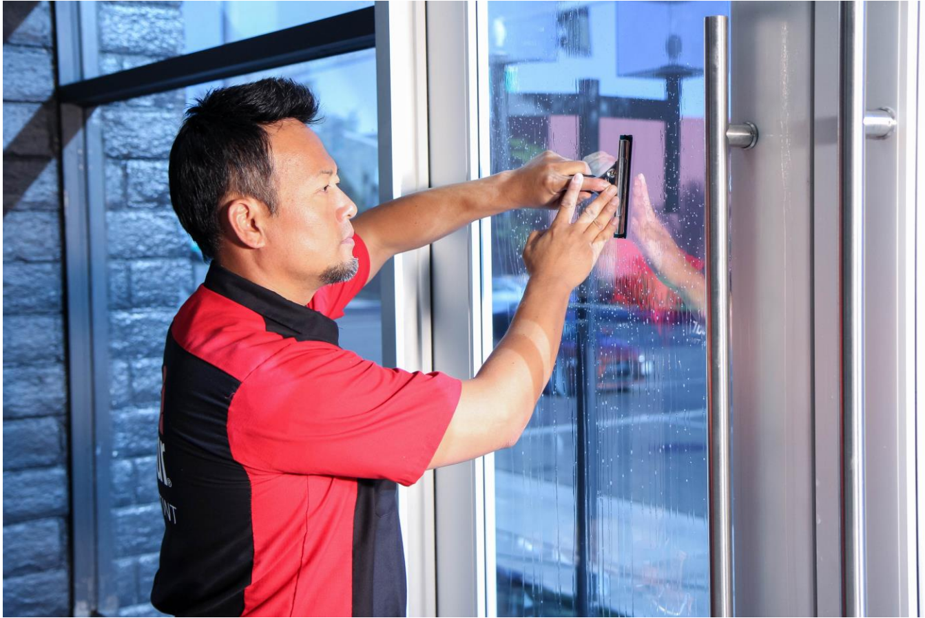
Figure 3. Installation of low-e applied film is similar to other plastic substrate applied films
