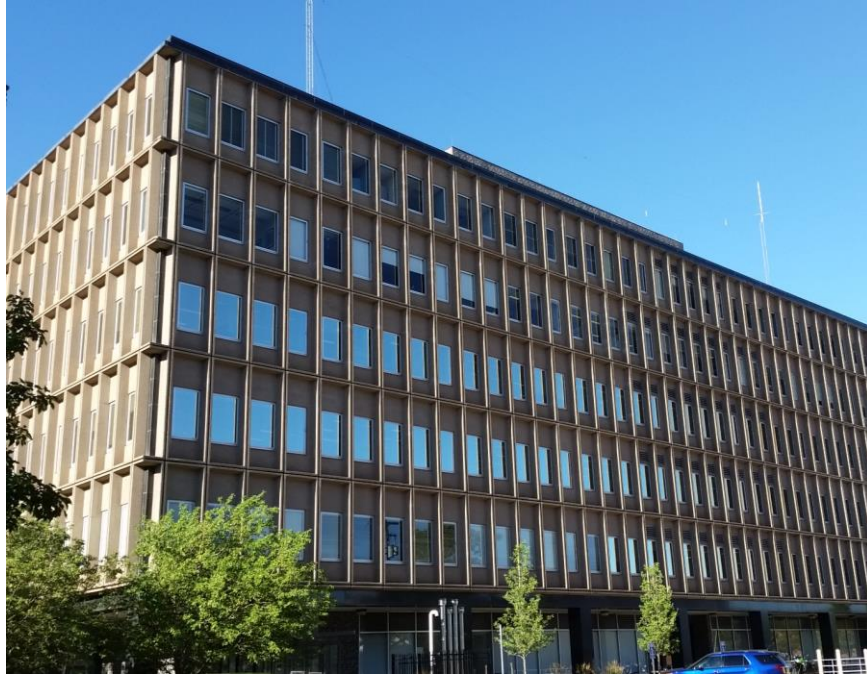
Figure 12. North facing side of the Hansen Building in Ogden, UT. The top two floors have no applied film. The lower floors have the low-e applied film installed and they appear more reflective from the exterior, providing a more uniform appearance.
