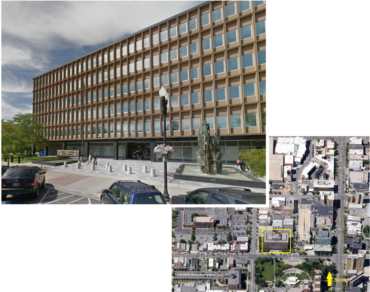
Figure 4. South façade of the Hansen Federal Building in Ogden, UT
