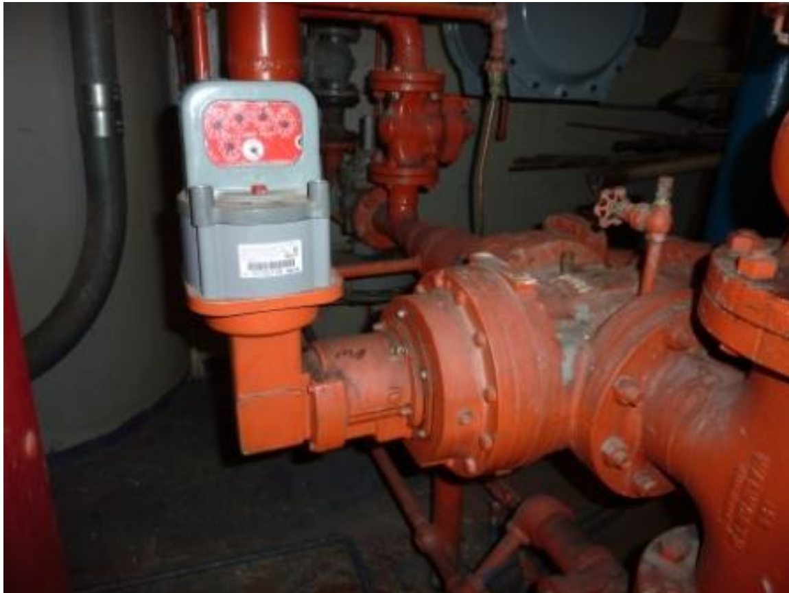
Figure 4: Photo of Natural Gas Meter located in the Basement that serves the Boiler Plant.
