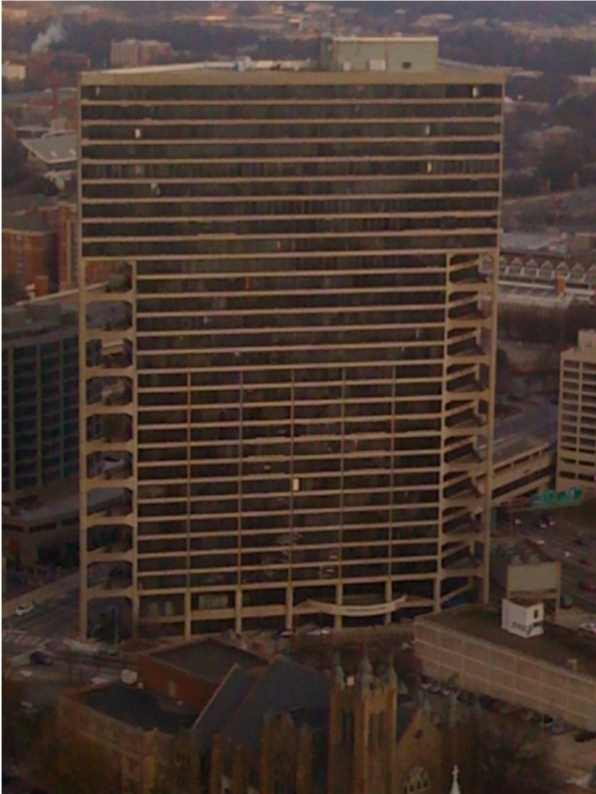
Figure 2: View of the Peachtree Summit Federal Building, Atlanta, Georgia.
