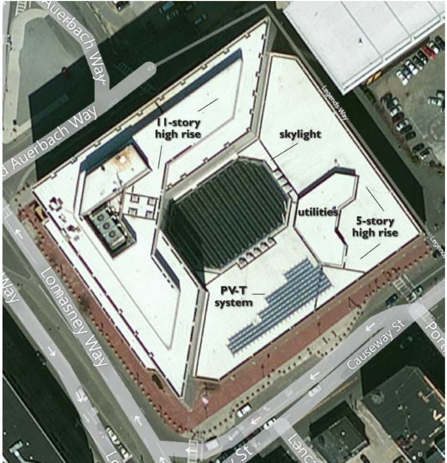
Figure 10. Aerial image of O'Neill Federal Building rooftop
