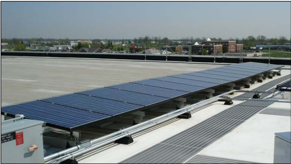
Figure 3: Medium Efficiency Crystalline PV Array, Laboratory PV systems, Bean Federal Center
