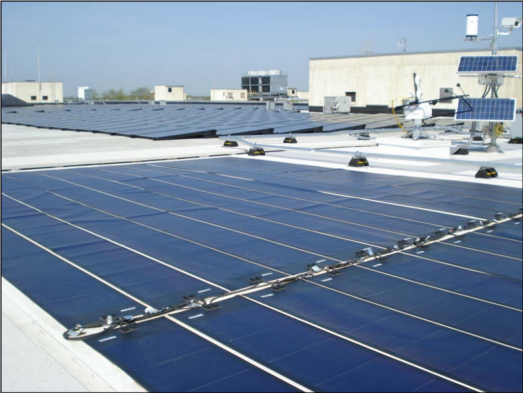
Figure 6: Thin-film a-Si Laminate PV Array, Laboratory PV systems, Bean Federal Center
