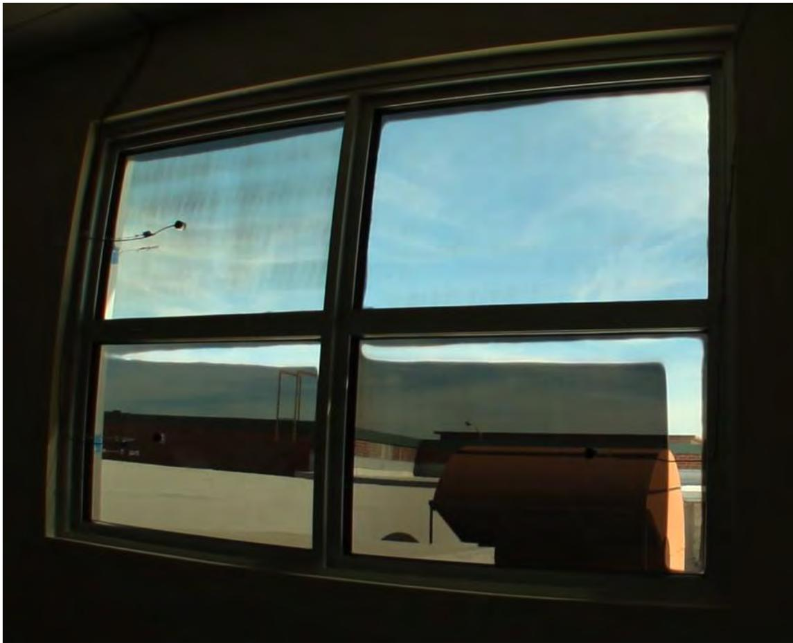
**Figure 14: Interior view of the right hand four panes from the infrared image in Figure 12. The lower panes are in thermochromic transition (horizontal mirror image flipped to match exterior IR). The upper panes are clear because they are shaded by the overhang outside the window. The upper and right edges of the lower panes are tinted due to shadowing by the frame and the middle and lower portions of the lower pane are tinted because the windows are in direct sun.**
