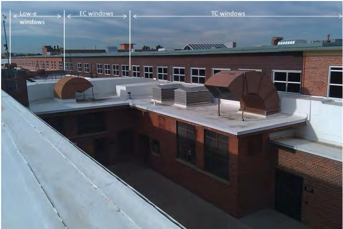
**Figure 2: Exterior view of the west façade showing the locations of the three types of windows. The low-e windows were installed in 2005. The electrochromic windows were installed in June 2011. The thermochromic windows were installed at the end of August 2011.**
