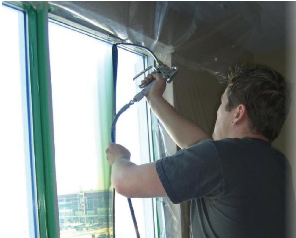
Figure 3. Installation of poured in place solar control film retrofit
