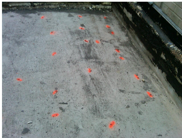
Figure 3. Fasteners from Old Roof, Marked for Grinding
