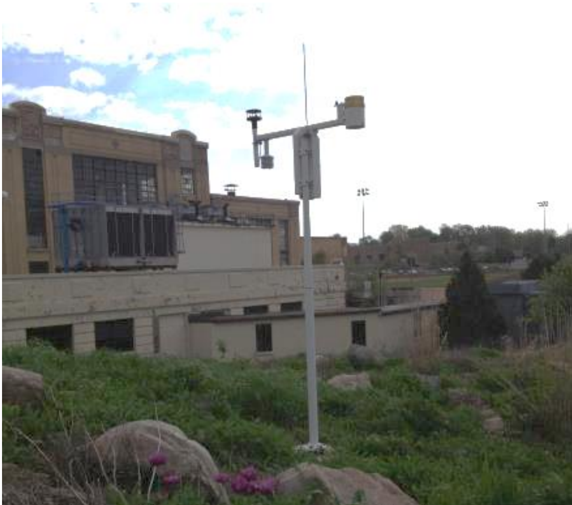
Figure 8. Weather Station at Hart-Dole-Inouye Federal Center
