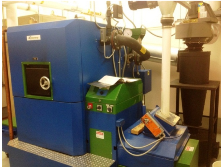
Figure 6: Boiler feed pipe
