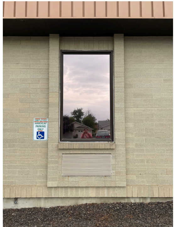
Exterior, typical window, 2021
