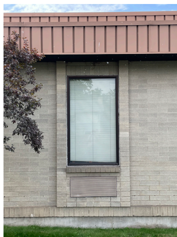
Typical bronze anodized aluminum window with brick surround and mechanical louver, 2021.
