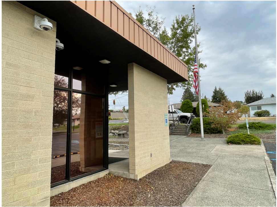
Exterior, view looking southwest at recessed entry and adjacent planter, 2021
