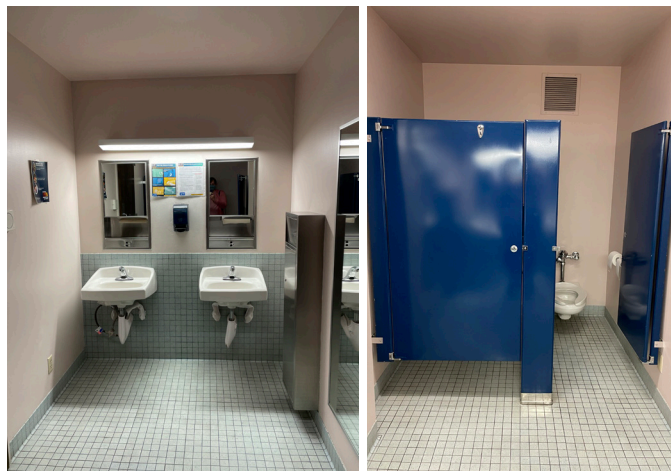
Original restroom finishes and fixtures, 2021.
