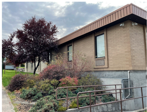
East elevation landscaping and ramp to basement from 17th Street sidewalk, 2021.
