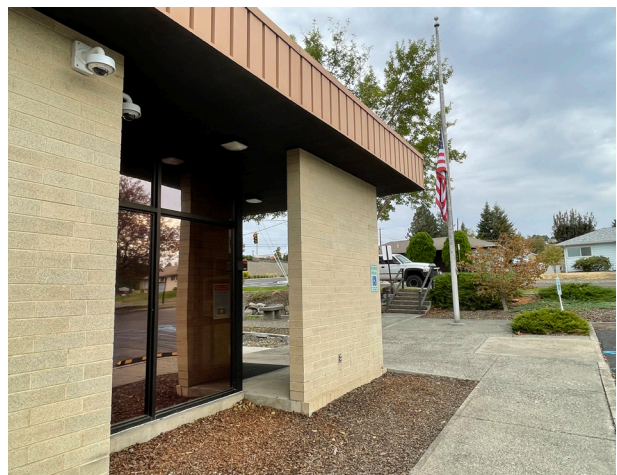
Entrance design features include floor to ceiling storefront glazing, independent brick support wall, Cedar slat soffit, metal panel fascia, and planter adjacent to the entry, 2021.
