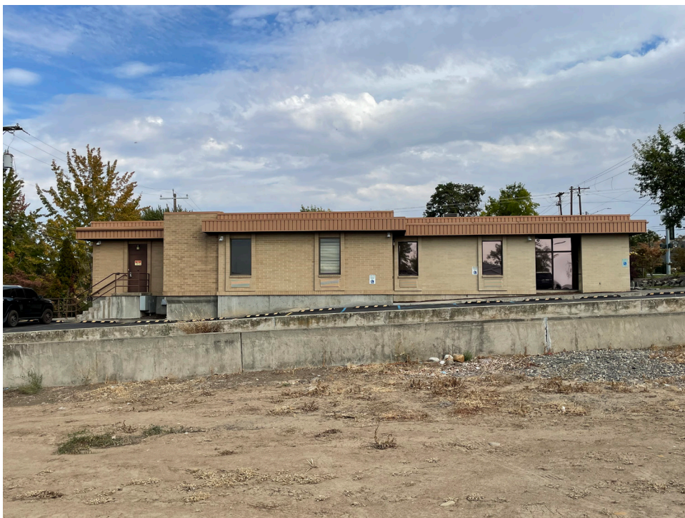
Exterior, west elevation, 2021
