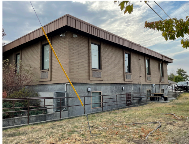
North elevation with ramp to basement entrance, 2021.
