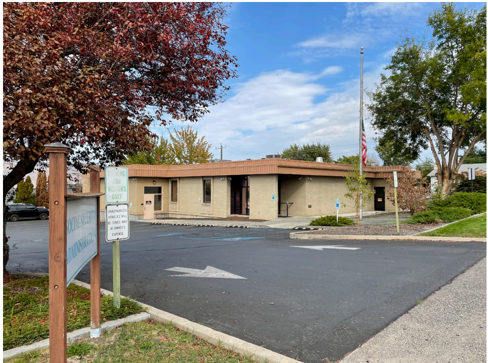
Exterior, view looking northeast at driveway and building entrance, 2021
