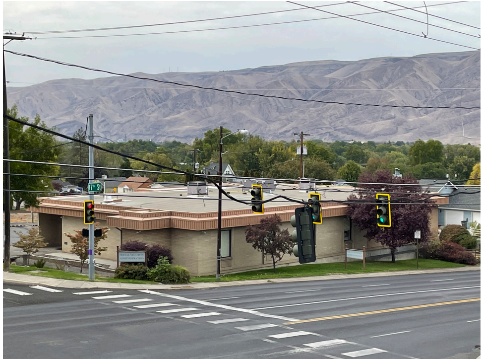
Exterior, view from adjacent shopping mall looking northwest, 2021
