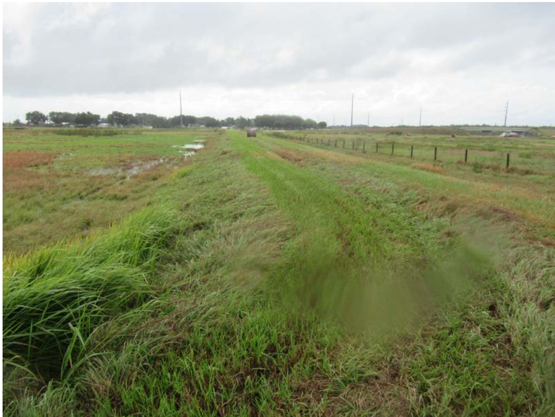
Photo 12: View of west side of onsite infiltration pond.
