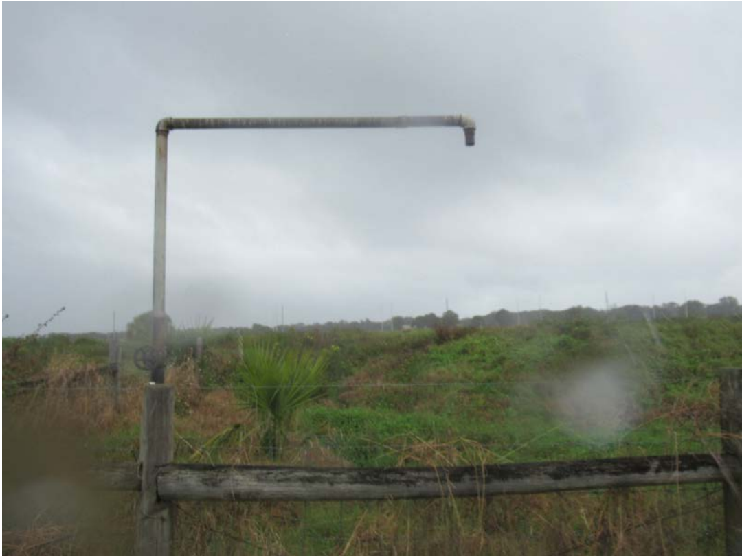
Photo 9: Overhead pipe at northwestern corner of the onsite infiltration pond.
