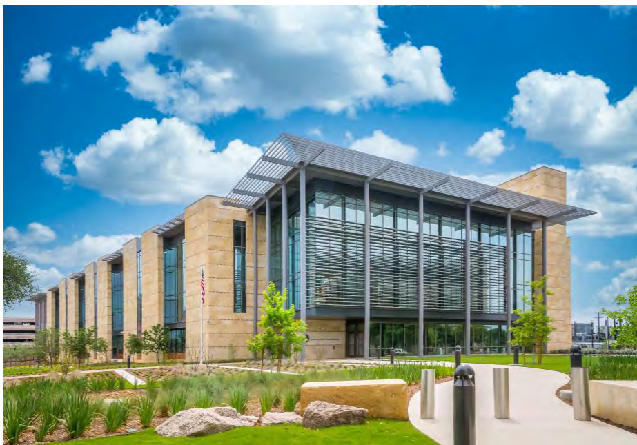
New Federal courthouse in downtown San Antonio stands 3 stories and includes a 235,000-square-foot building with 8 courtrooms and 13 chambers (Photo credit: Daniel W. Torres Photography)
