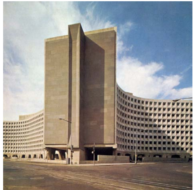
The Robert C. Weaver Federal Building, Washington, D.C. Breuer, Marcel, 1968, photographer
