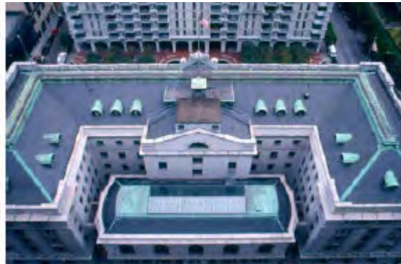
Photo: U.S. Custom House Roof. Credit: GSA c.2000 (GSA 2008).
