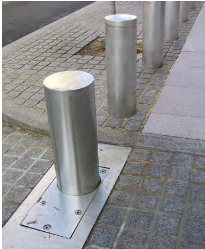
Pop-up bollards can provide perimeter protection, while permitting controlled access for emergency or delivery vehicles (left). Although clamshell-style barriers are less costly and require shallower mounting depths, they are uniformly unattractive and, in most cases, should be avoided or screened where possible (right). A better option may be a turntable type system (see page 47).
