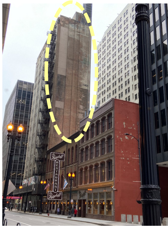
Figure 3.2-4. Picture Taken on Adams Street showing West Elevation/Face of 202 South State Street (circled)
