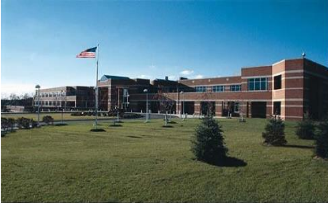
VA DAYCARE BUILDING – PHILADELPHIA, PA
