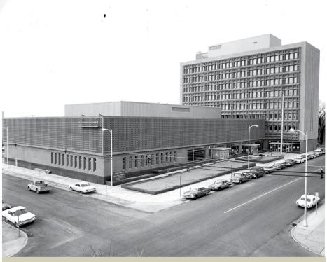
Built in 1964, the Joseph C. O'Mahoney Federal Building/ Post Office (FB/PO) was designed in the Formalist style and is a distinctive building in downtown Cheyenne. The FB/PO has two structures. The post office is a two story plus basement structure that is attached to an eight story tower that projects up from the north end of the building. The building is clad with precast
