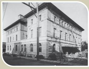
granite and limestone. The first through third floors are clad with ashlar limestone which is finished differently at each floor.
