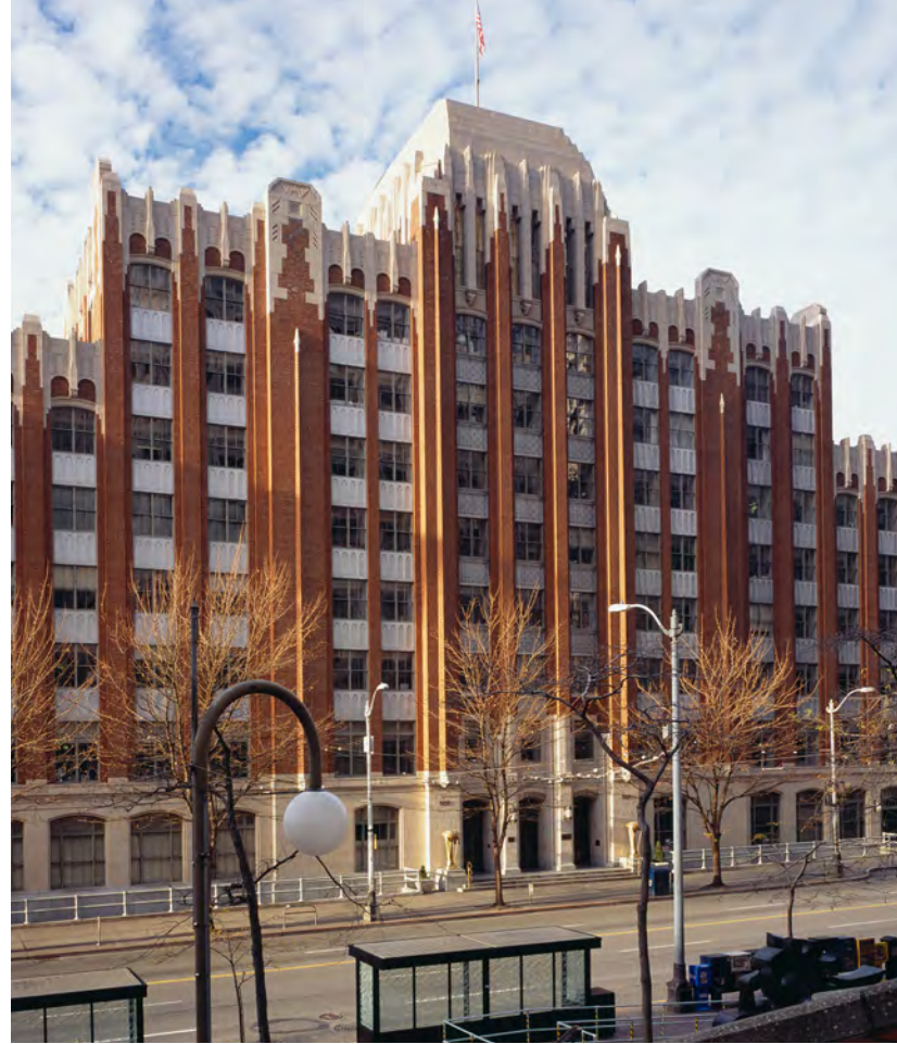
MONTHLY LASER SCANS AT GSA'S 1932 FEDERAL BUILDING IN SEATTLE ARE NOW BEING USED TO ASSESS EFFECTS OF TUNNEL DRILLING FOR CONSTRUCTION OF THE SEATTLE'S SUBTERRANEAN HIGHWAY 99, SCHEDULED TO OPEN IN 2019.
