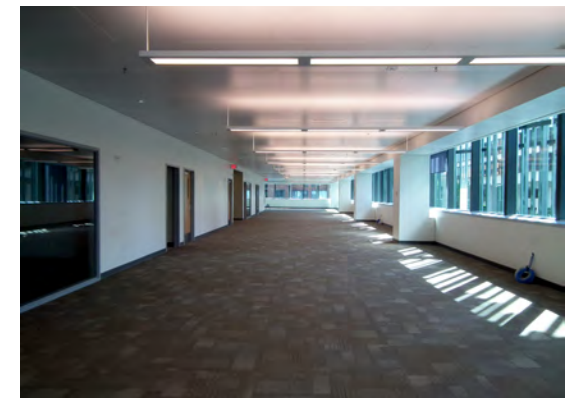
Image: Radiant ceiling panels
