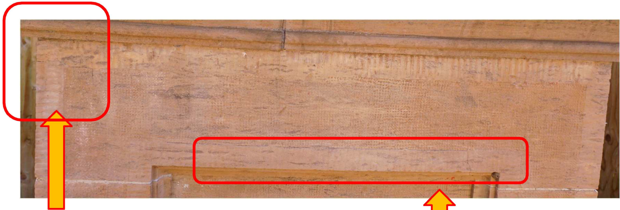
Material cracking, depth unknown, potentially continuation with cracks at adjacent face of stone.
