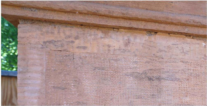
Material cracking, depth unknown, potentially continuation with cracks at adjacent face of stone.
