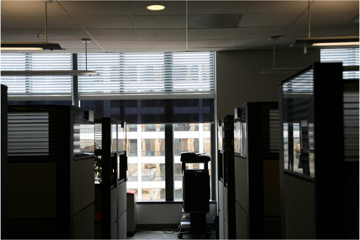
Figure 11. Indoor view of the southeast-facing open plan office area in the Oakland Federal Building with automated upper louvers and manually operated lower GS shade. The GS shade is partially lowered in this photograph. Workstation partitions were 5.5 ft. high.
