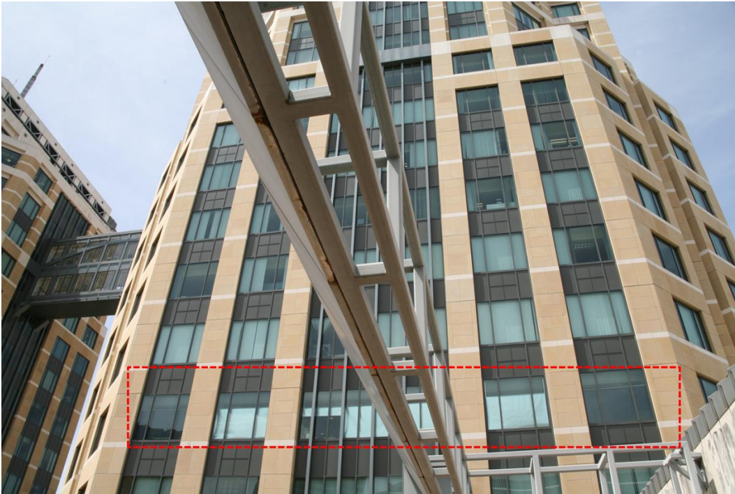
Figure 6. Outdoor view of the Oakland Federal Building with manually operated GS (bright white) and GG (dark gray) shades on the southeast facade.
