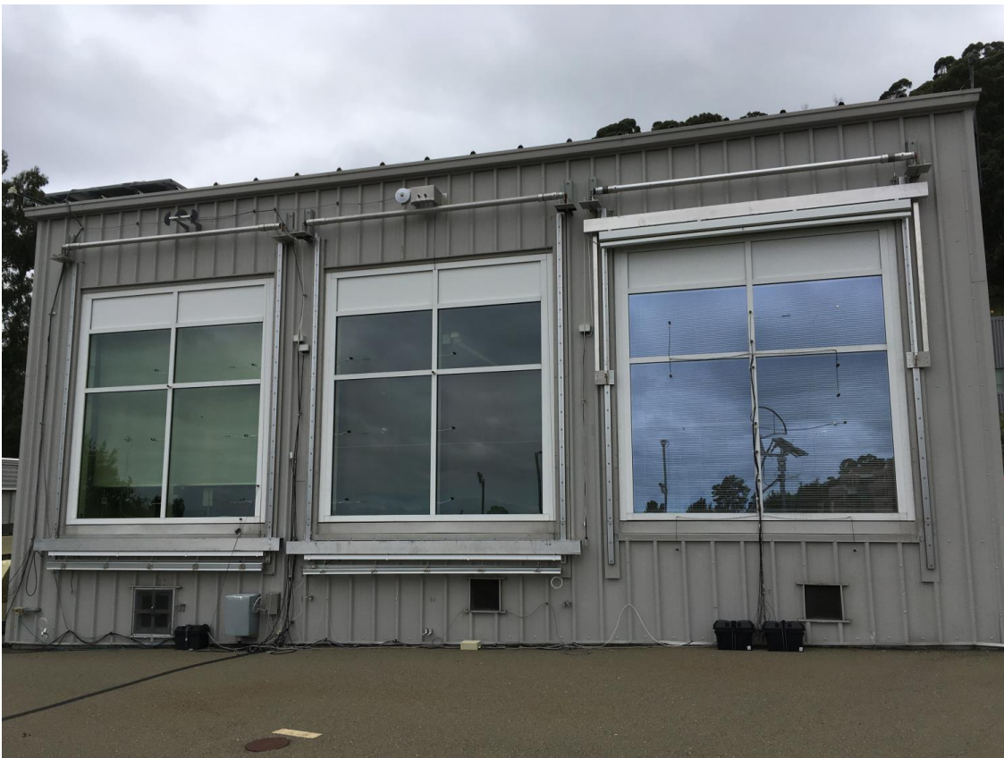
Figure 14. Exterior view of the LBNL Advanced Windows Testbed (B71T). The auto-GG shade is shown in the middle test chamber. A conventional roller shade (left) and venetian blind (right) are shown in the other two test chambers.
