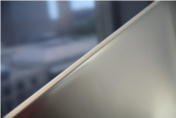
Figure 13. Close-up view of the lower GS roller shade in the Oakland Federal Building: upper area shows the slightly diffused view through the film and the lower area shows the slightly textured reflective back side of the same film.
