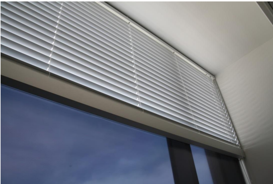
Figure 12. Close-up view of reflected daylight off the upper white louvers in the Oakland Federal Building.
