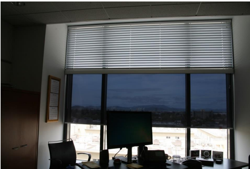
Figure 10. Indoor view of the northwest-facing office in the Oakland Federal Building with manually operated upper louvers and manually operated lower GS shade. The GS shade is partially lowered in this photograph.
