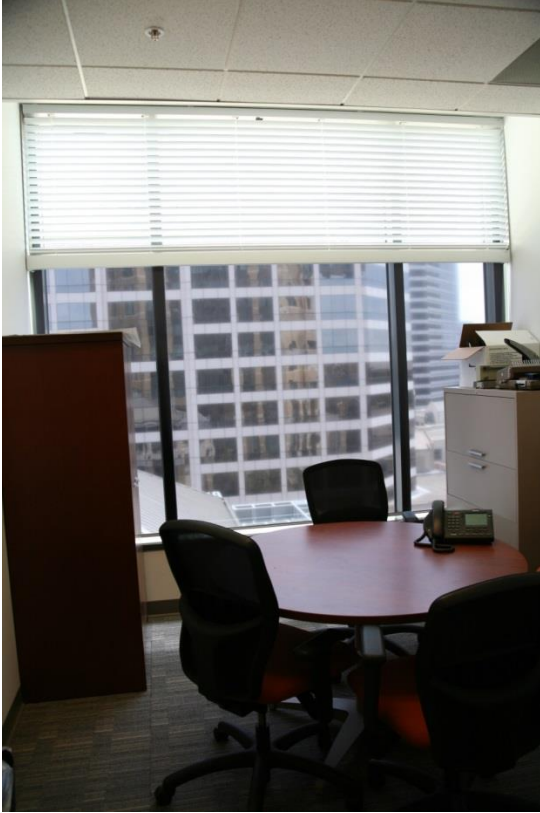
Figure 9. Indoor view of a southeast-facing office in the Oakland Federal Building with automated upper louvers and lower manually operated GS shades on the southeast facade. The GS shade is fully lowered in this photograph.
