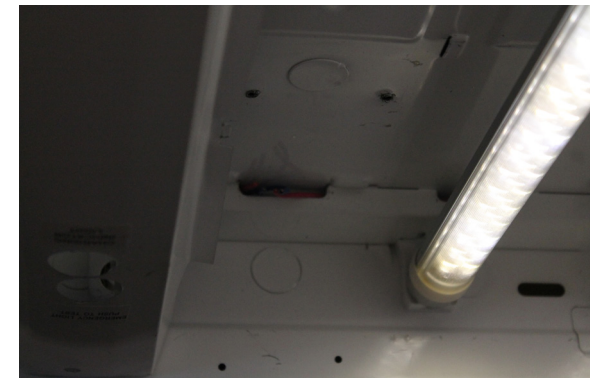
Low-quality TLEDs show each row of LEDs in the tube and result in a “pixelated” appearance. Photo credit Michael Myer, PNNL
