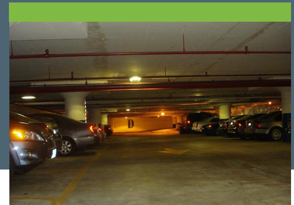
Integral occupancy sensor in parking garage luminaire increases output when motion is detected. Photo credit Akoya, U.S. DOE
