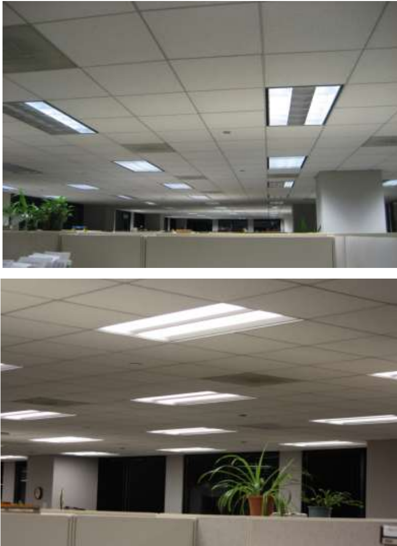
Figure 20: Pre (top) and post (bottom) retrofit ceiling photographs at Metcalfe
