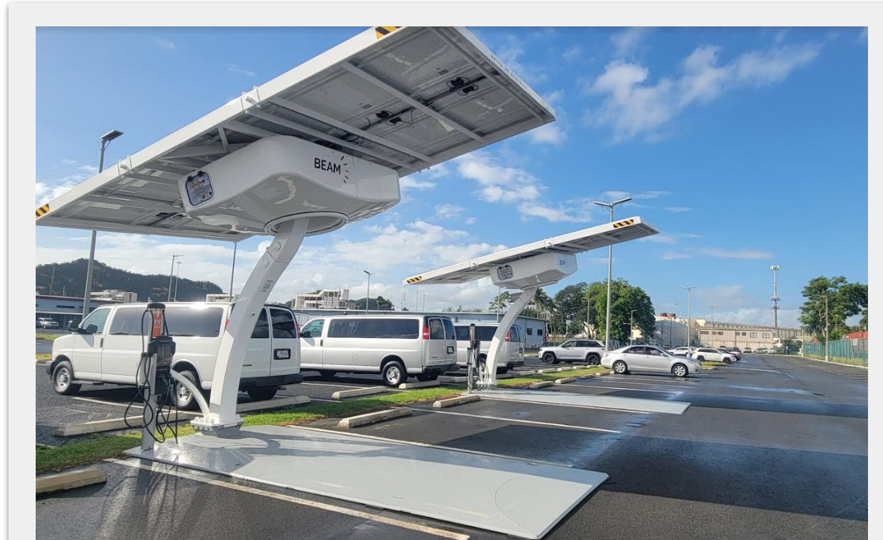
Army Corps of Engineers - Solar Install in Galveston, TX
