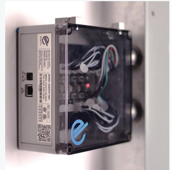
Full-Panel Submeter Photo credit Enertiv
