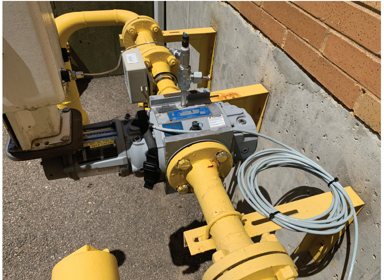
Strap-on Submeter with Turbine Gas Meter. Photo credit Vata Verks
