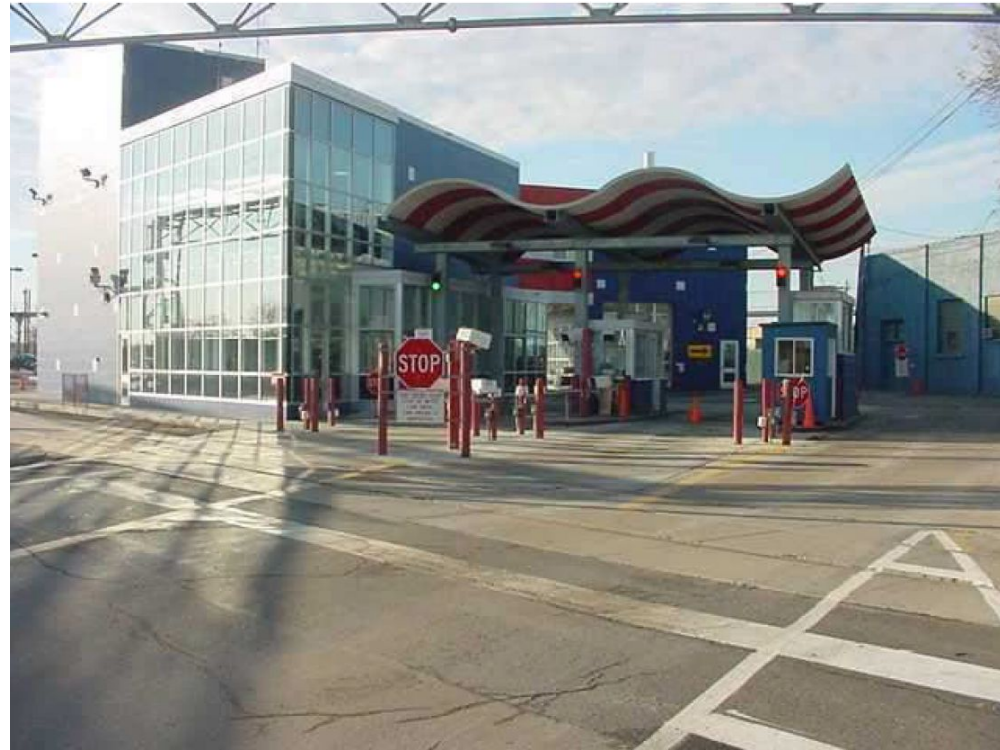
International Falls Land Port of Entry (LPOE), Minnesota
