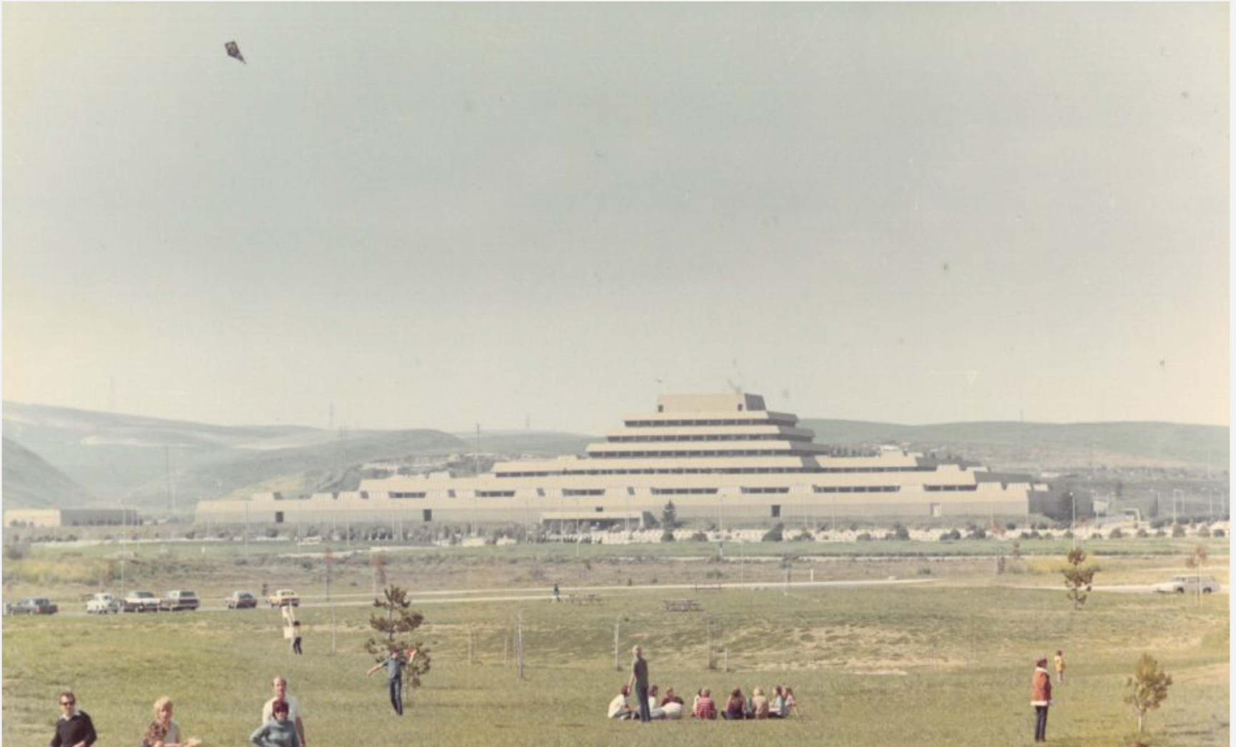
GSA Photo ca. 1971
