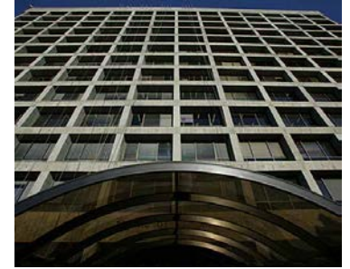
Figure 5 – Building 67 (Source: Centerre Construction)
