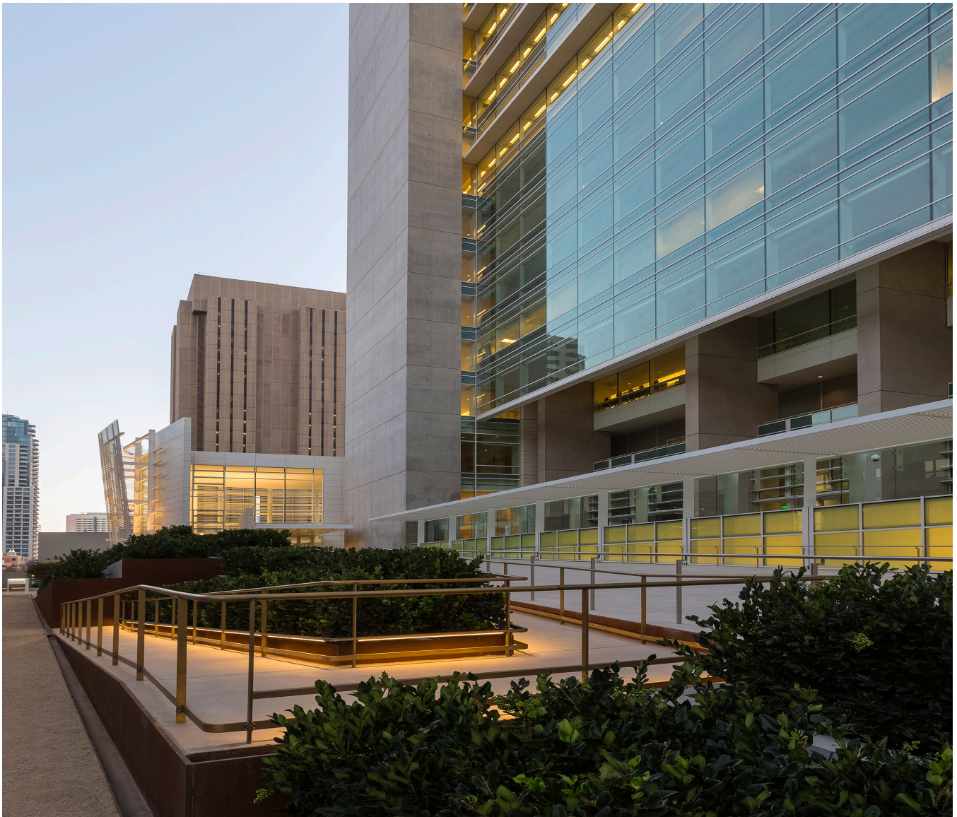
Entrance Ramp - United States Courthouse Annex, San Diego, California
