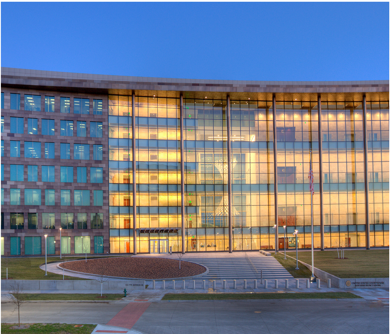
Approach to Main Entrance - United States Courthouse, Cedar Rapids, Iowa
