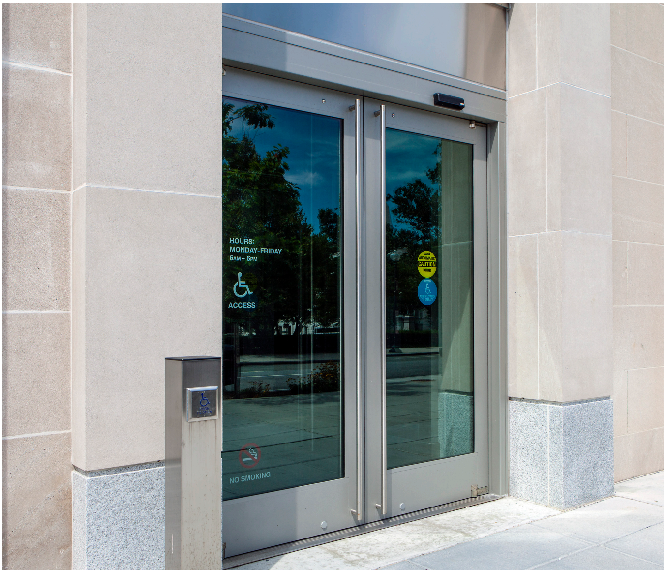
New E Street Entrance Doors - GSA Headquarters, Washington, DC
