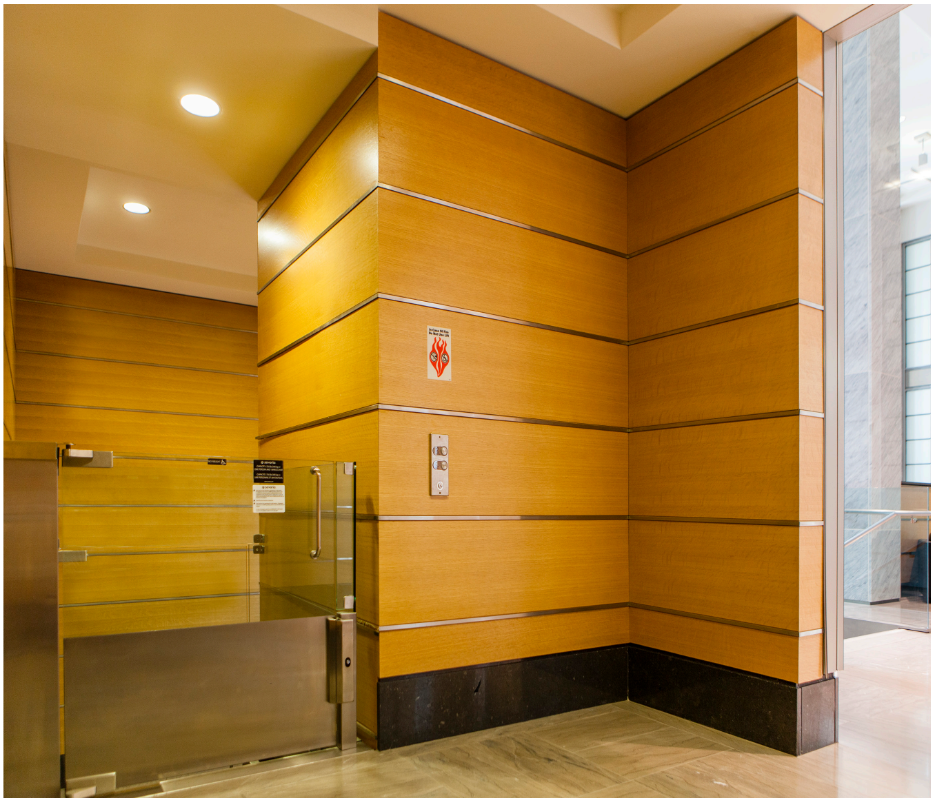
New E Street Entrance/Ground Floor Wheelchair Platform Lift - GSA Headquarters, Washington, DC
