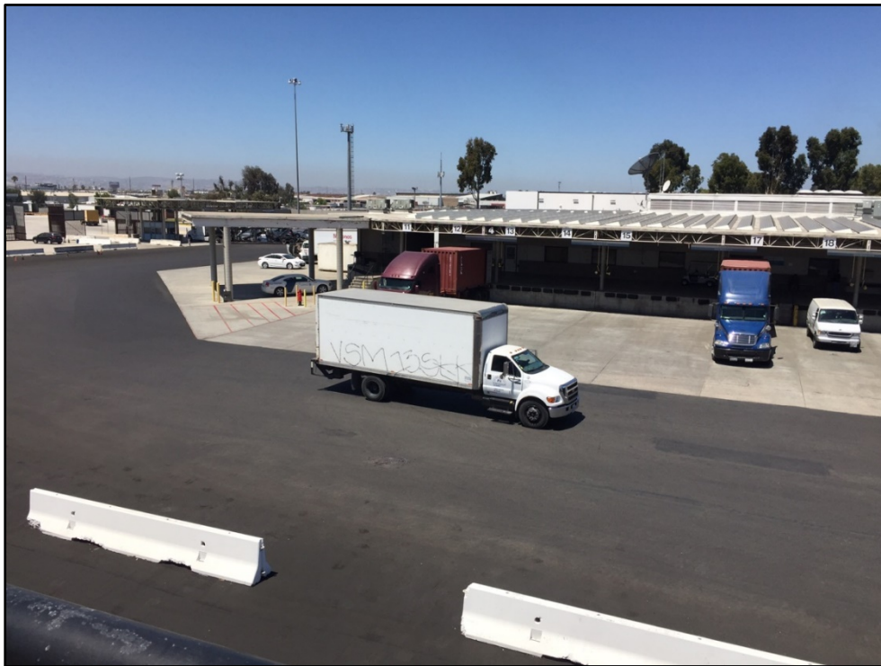
Figure 3.10-1. View of Existing Otay Mesa LPOE Commercial Import Building
