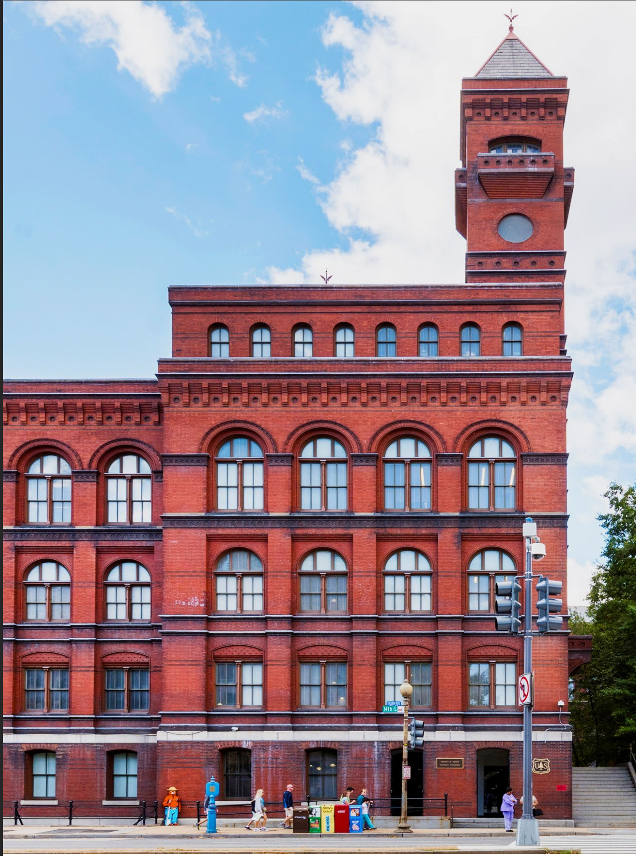
Figure 4: Sydney R. Yates Federal Building Washington, DC
