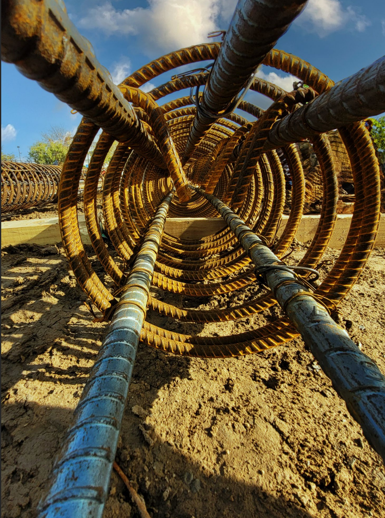
Figure 13: U.S. Courthouse Structure Greenville, MS
