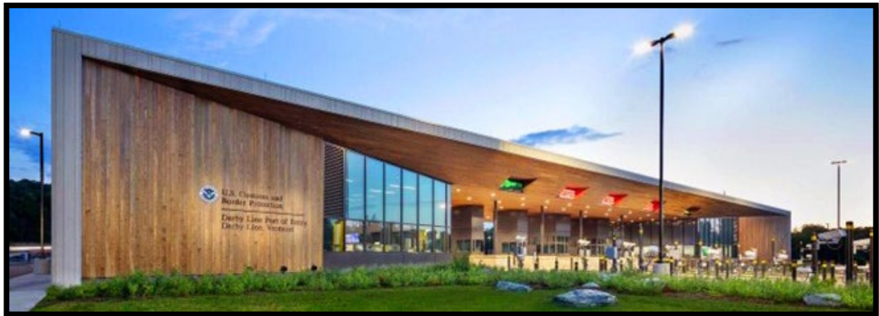
Figure 10: Land Port of Entry Derby Line, VT
