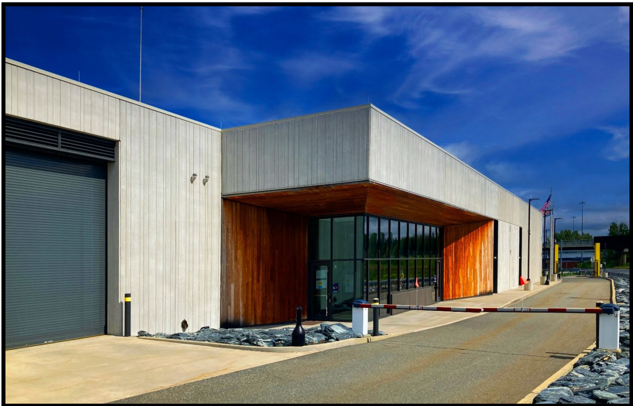
Figure 25: Land Port of Entry Derby Line, VT
