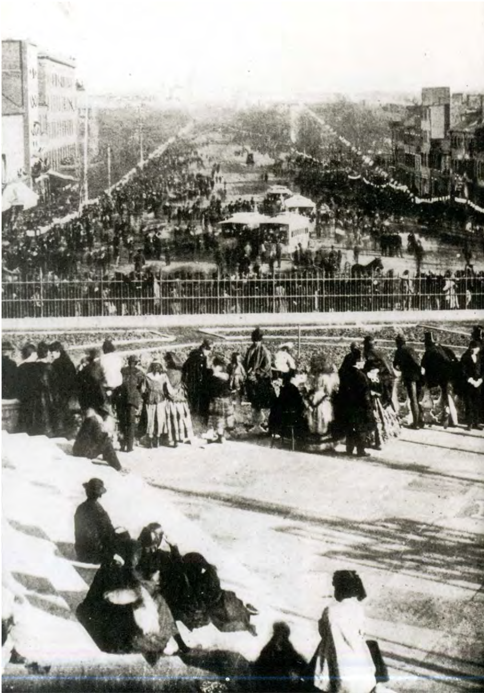
Fig. 6: The city celebrated the installation of the new wooden pavement with a two-day carnival held February 20 and 21, 1871, during which President Grant proceeded down the avenue in his carriage (Highsmith)
