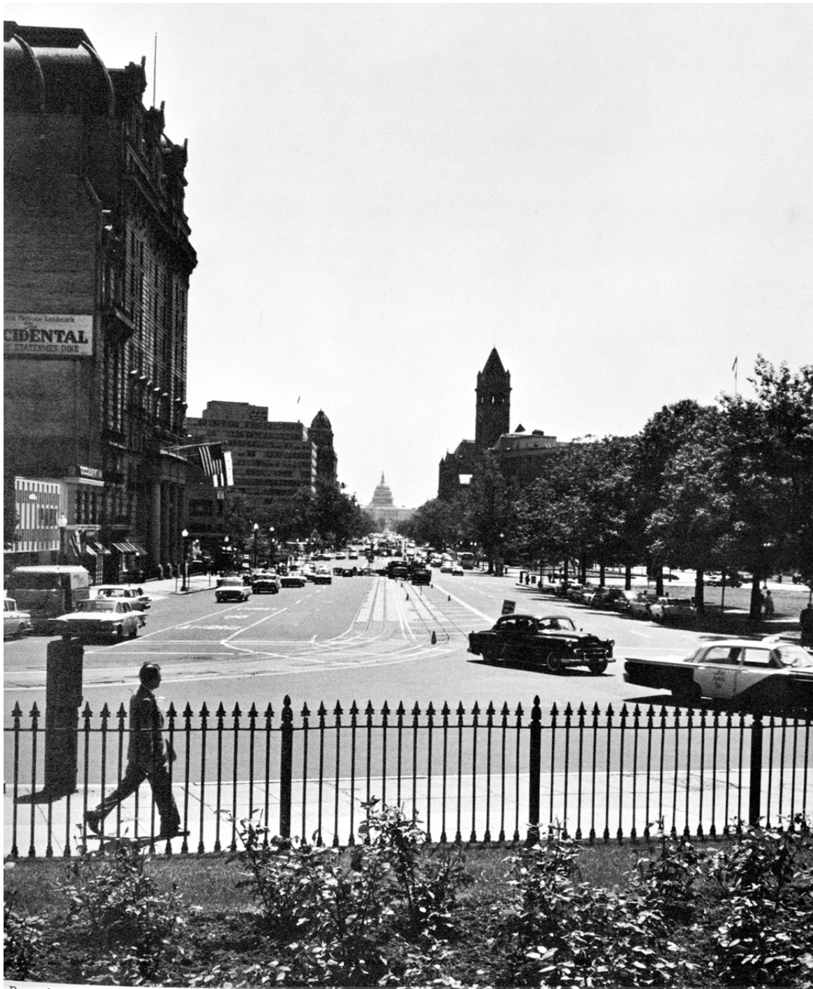
Pennsylvania Avenue seen in 1962 from Treasury Place, before removal of car tracks.
