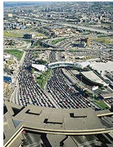
Aerial view of San Ysidro Border Crossing, San Ysidro, CA
