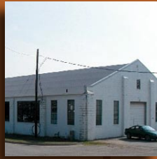
PMD Center Warehouse Oklahoma City, OK
