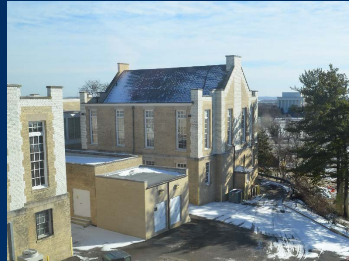
Southwest Ward, North Elevation
