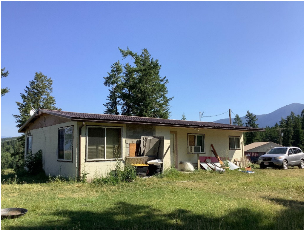
Figure 6. 147 Trading Post Road. Oblique view of south and west facing façades.
