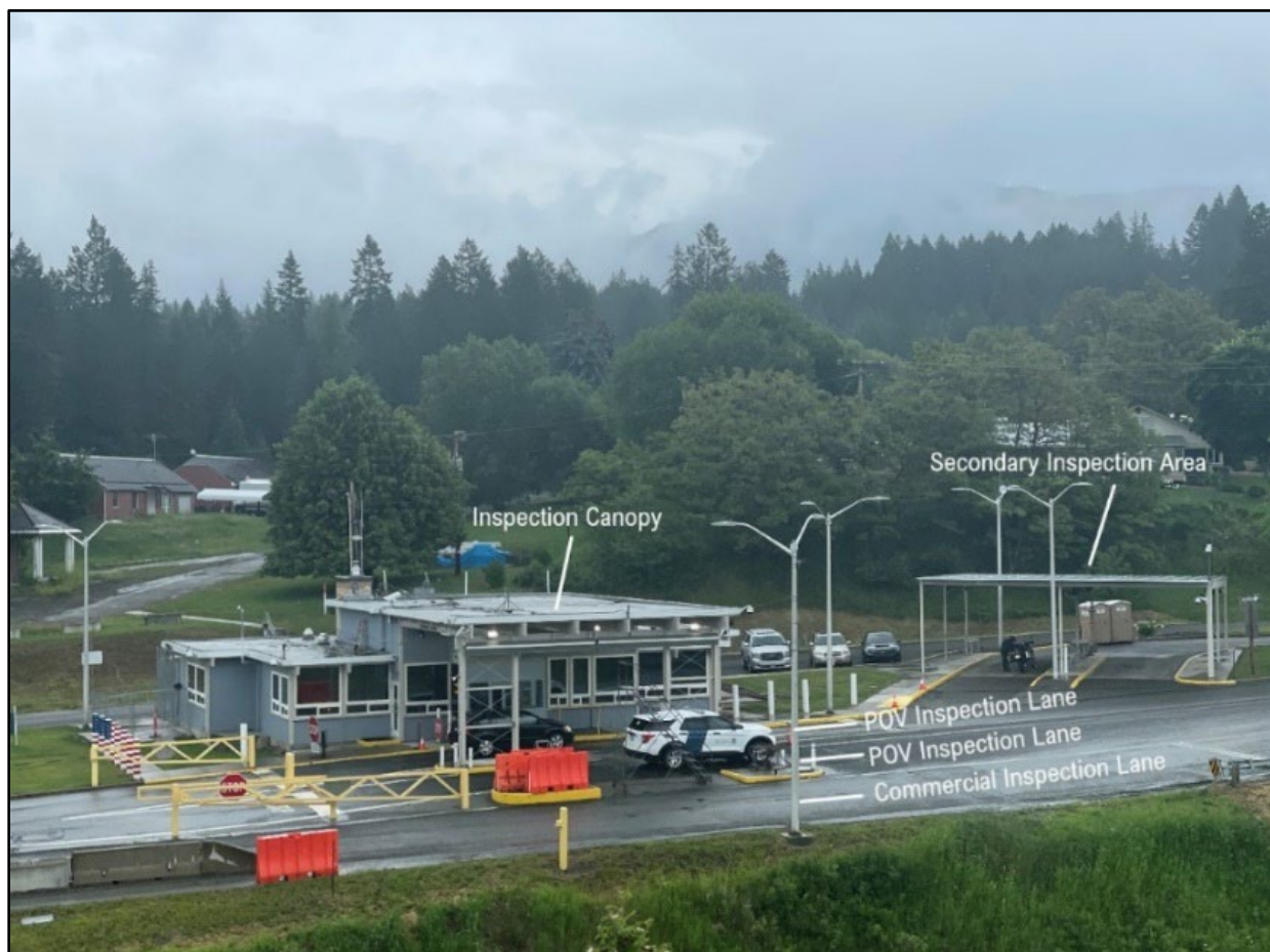
Figure 1.2-3. East-facing View of Inspection Lanes with Inspection Booth and Canopy Accessible Only to Inner Lane
