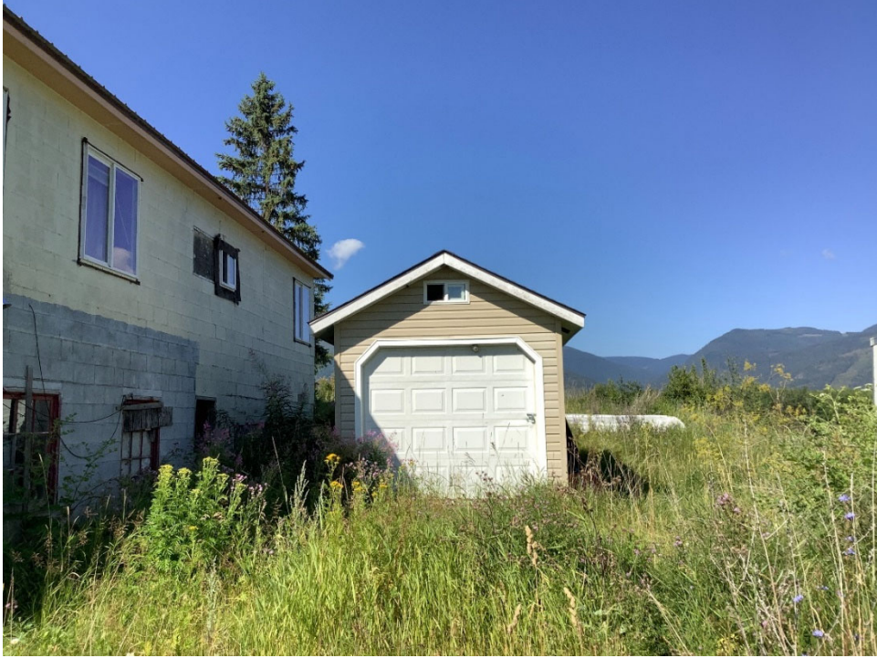
Figure 13. Shed, adjacent to the north of 147 Trading Post Road. View toward west.
