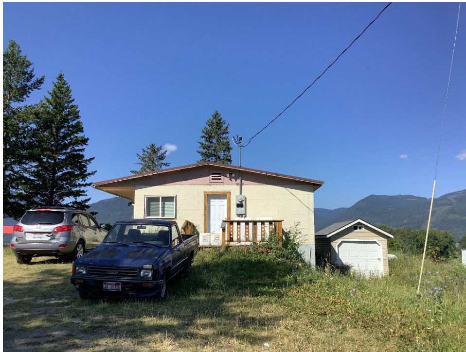
Figure 9. East facing façade of 147 Trading Post Road. View toward west.
