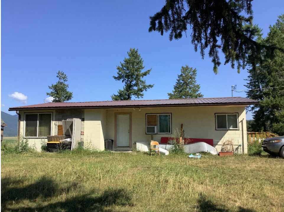
Figure 7. Primary façade of 147 Trading Post Road. View toward north.
