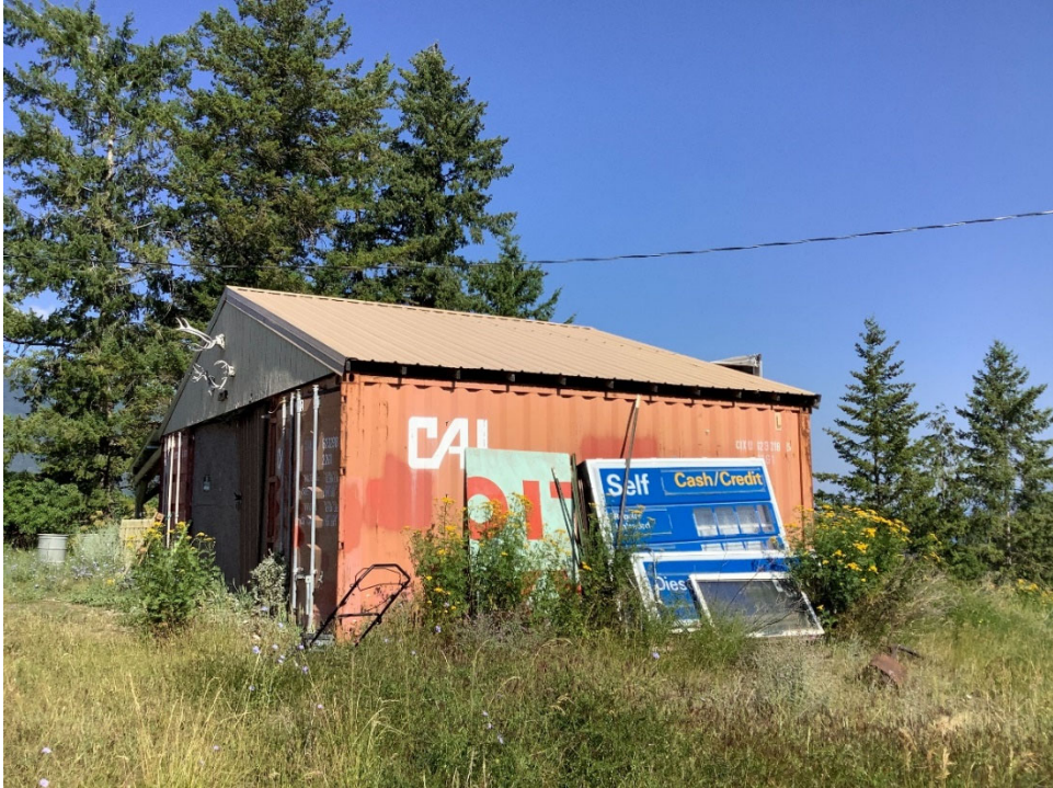
Figure 14. Oblique view of larger shed on the eastern side of the property. Oblique view of southern and western facing façades, view toward northeast.
