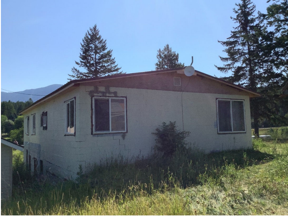
Figure 11. East facing side façade of 147 Trading Post Road. View toward west.
